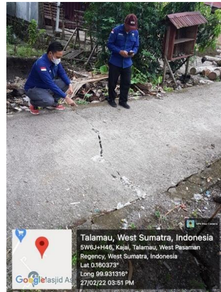
Fig.12. Ground failure at residential area Kajai Village
