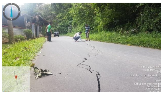
Fig.9. Ground Cracking at Talu Village
